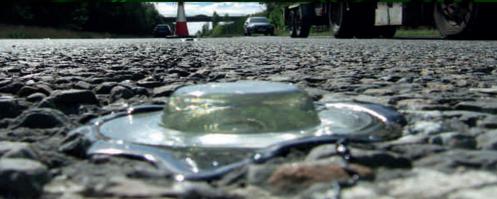
The Siglite glass road stud is a heavy duty road marker, designed for use in all highways, including motorways, trunk roads and urban locations. It has a good level of retro-reflectivity, which is visible across a very wide approach angle and which is retained over along period of time, qualifying for the highest R1 retroreflectivity rating. Siglites are made from fully tempered long life glass and withstand high traffic volumes.
