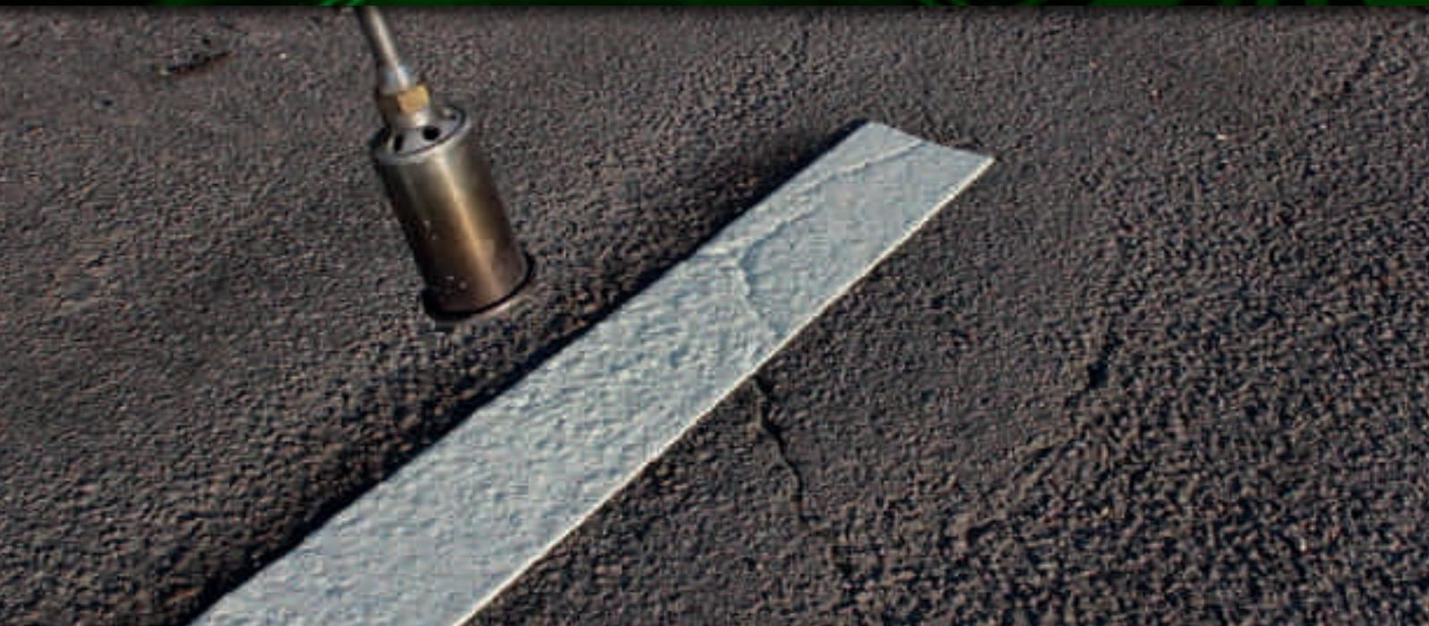
MagmaLine Plus is a roadmarking line product made from preformed thermoplastic, used to lay permanent lines onto asphalt surfaces. It is easily laid, durable and meets Highway standards, without the call-out costs associated with screed applied thermoplastic lines. It has an advanced Plus formulation which retains flexibility even in cooler conditions; this overcomes a major drawback with other brands and enables work to continue through winter months.
