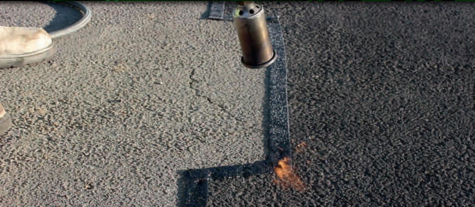
ThermaBand Plus is an overbanding product made from thermoplastic, which is used to seal joints in asphalt surfaces, preventing water ingress and associated frost damage. It has an advanced 'Plus' formulation which retains flexibility even in cooler conditions and has an anti-skid treatment impregnated into the surface.
